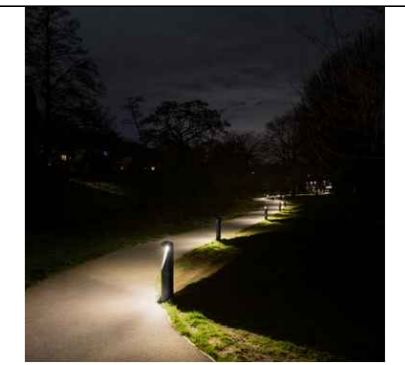
Example bollard / low level lighting with zero upward light at low lighting level with a low mounting height.
